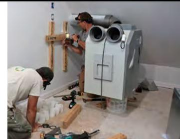
**Taming the tubes.** One of the carpenters cuts the Zehnder duct tubes to length before connecting them to the manifold.
