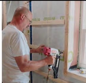
**Sealed on the inside.** The *Intello Plus* acts as both an air barrier and netting for the blown-in cellulose insulation, and the strapping ensures flat drywall.
